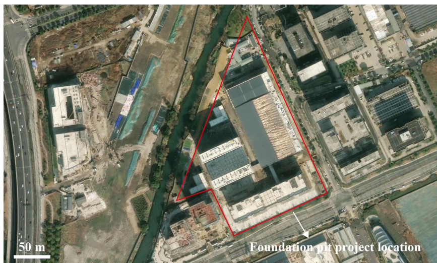
Figure 1. Surrounding environment of foundation pit.
