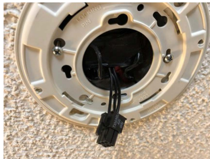
Figure 9. Device Installed in Ceiling. Once the smoke detector is installed in ceiling, there is no way to find the hardware in plant since they are hidden inside the ceiling.
