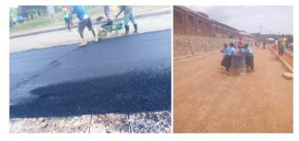
**Figure 2.** Lack of safety measures to road Workers for asphalt and land surveying activities and road users like children.
