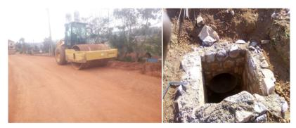
**Figure 12.** Lack of Adequate Signs to warn parked Machine at Karama Road and a manhole under construction at Akagera Road.
