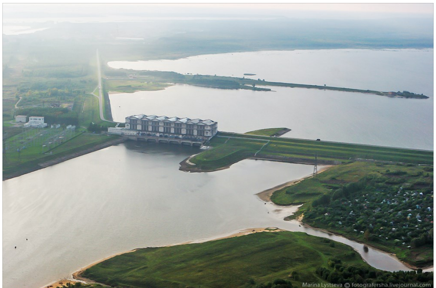
Figure 17. Rybinsk hydroelectric dam. Photo Credit: Megaconstruccion.es.
