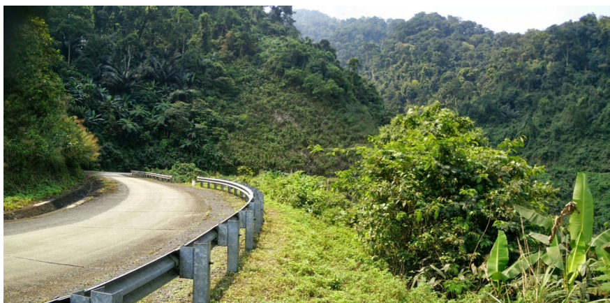
Figure 26. Ho Chi Minh two-lane road is being widened to become an eight-lane Ho Chi Minh highway.
