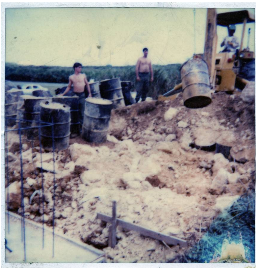
Figure 11. Repacking herbicide barrels and recovering buried barrels leaking into the ground. Reprinted with permission from Editor of the Open Journal of Soil Science.
