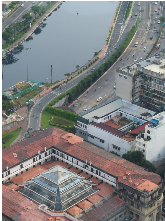
Figure 7. Thiem Tunnel entrance near a tributary of the Saigon River. The six lane road disappears under a green tree line in the center of the photograph.
