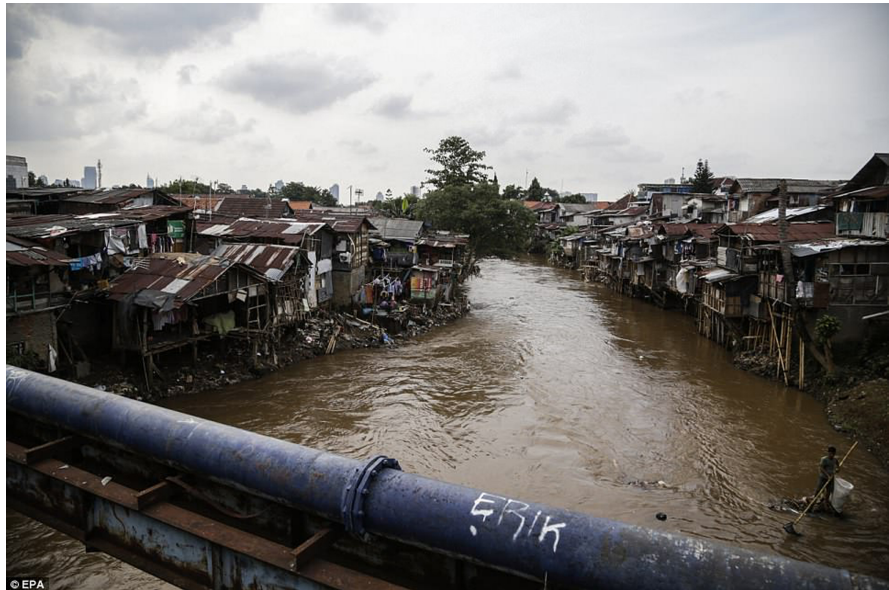
Figure 10. Trapped water flooding at Jakarta drainage ditch, which is lined with home sites. The ditch was dredged to improve the flow of drainage water. Courtesy of the Jakarta Post.
