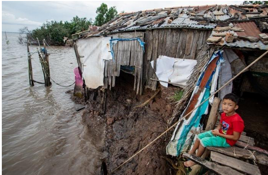
Figure 15. Vietnam shore erosion along the Mekong River. The house is failing into the river. Credit Line: Courtesy of DTi News.
