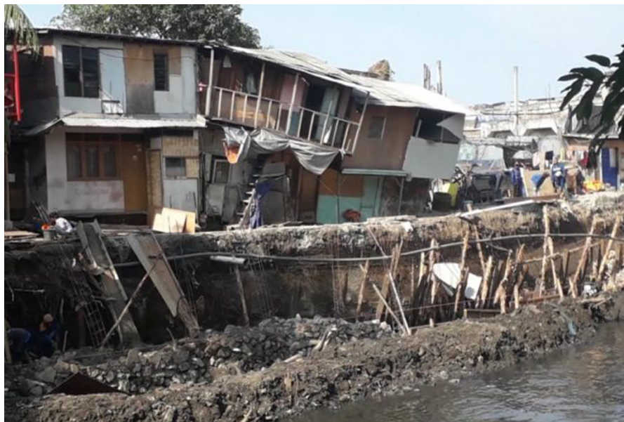
Figure 11. River bank landslides in Jakarta. Credit Line: Courtesy of the Jakarta Post.
