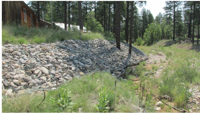
Figure 34. Gully erosion control structures on tributary streams of the Upper Rio Grande.
