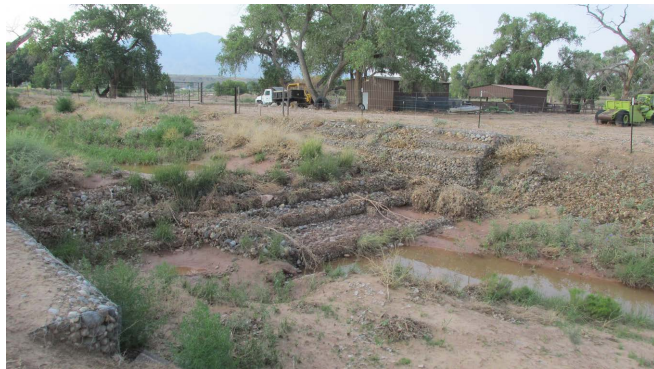
Figure 35. Stream bank erosion control structure on Rio Grande tributary streams.
