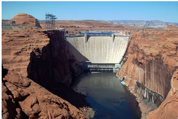
Figure 24. Glen Canyon Dam and the Colorado River canyon.
