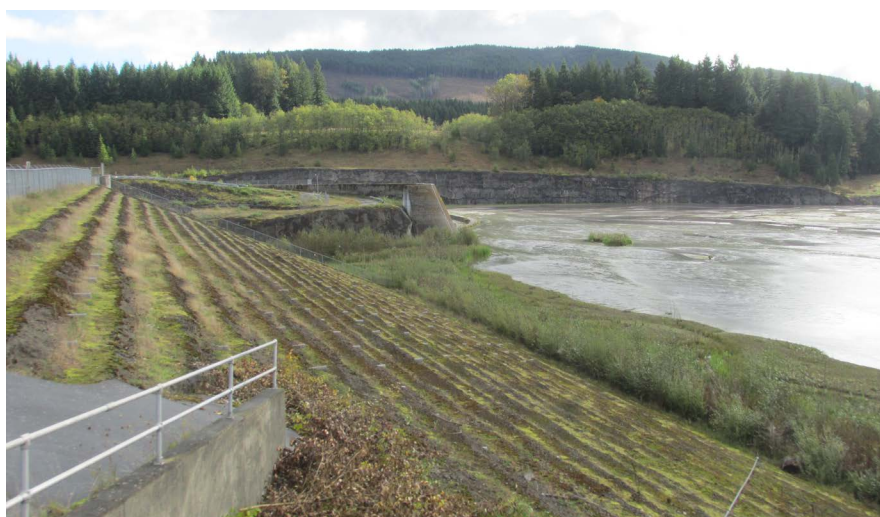
Figure 21. The Mount St. Helens mudflows reached the Columbia River and adversely affected navigation so Congress authorized the United State Corps of Engineers to block the sediments on the North Fork of the Toutle River.
