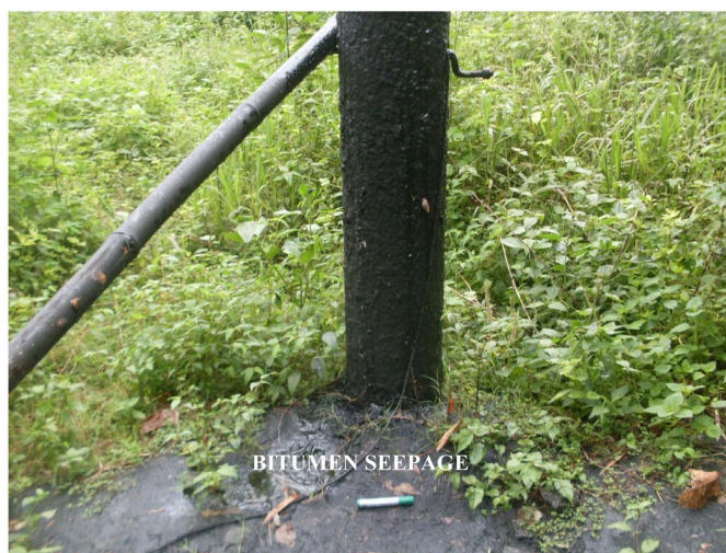
Figure 5. Picture of the bitumen well casing at Agbabu.
