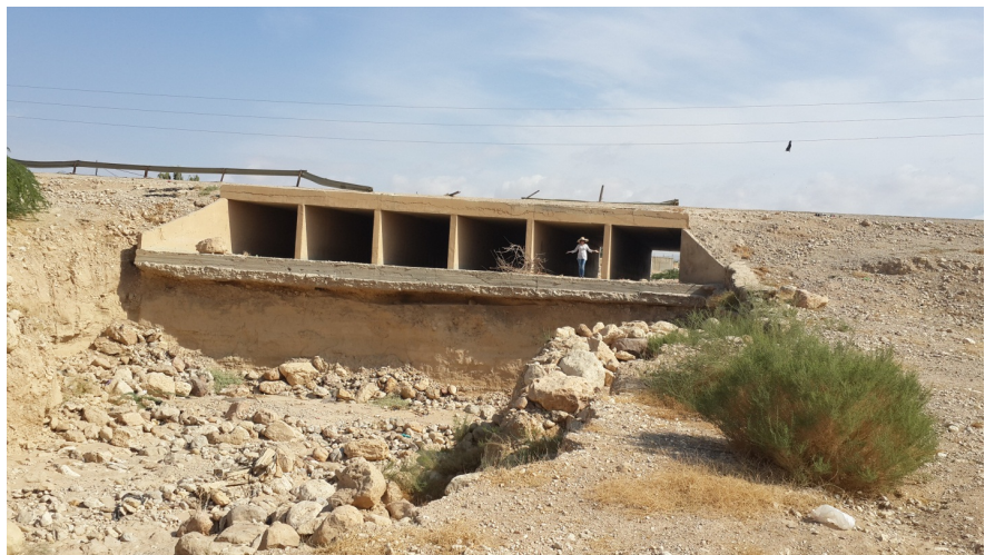
Figure 11. Severe undercutting and erosion affecting the foundation of the main Dead Sea road culvert, by now threatened to collapse.
