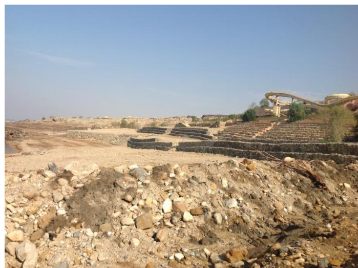
Figure 12. Gabion walls and terraces as a solution to the erosion problem in the newly formed terraces' areas which have been evacuated of Dead Sea water.
