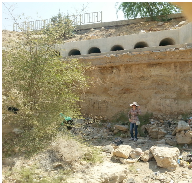
Figure 10. Head-ward erosion along one of the wadis in the study area. It has reached the main road built along the Dead Sea, which shore lies now at around 600m west of that main road. The height (thickness) of eroded materials is around 5 m and erosion has started to excavate the rocks underlying the main road.
