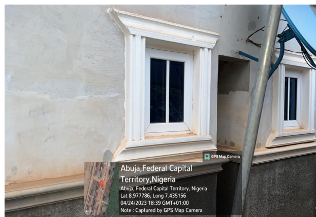
Plate 2. Shaded window at Pent Estate. Source: Field Work, 2023.
