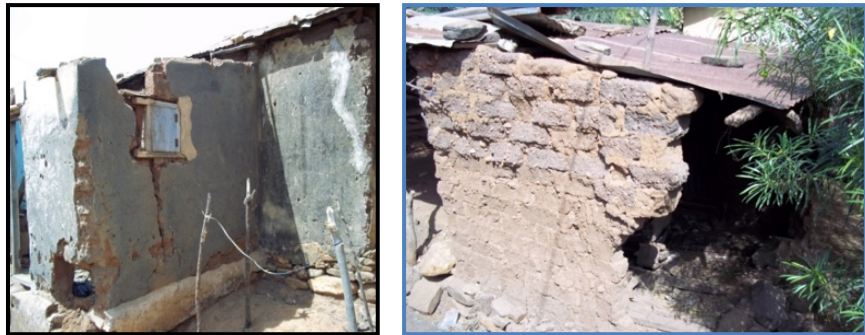
Figure 4. Typical examples of the ruin of earthen constructions.
