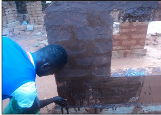
Figure 17. Application of the bonding layer.
