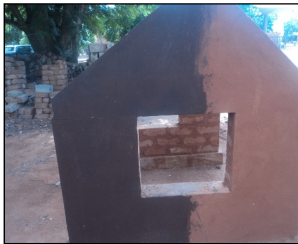
Figure 21. Wall after application of the protective layer.
