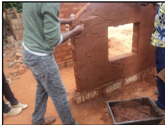
Figure 19. Application of the body of the coating.
