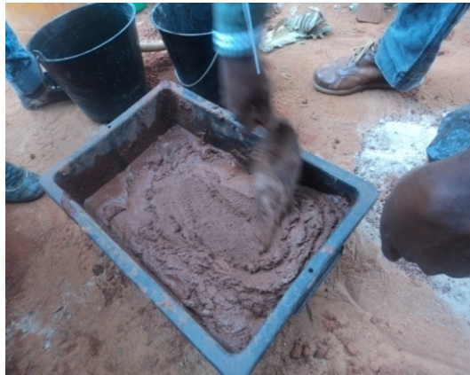
Figure 18. Preparation of the body of the coating.
