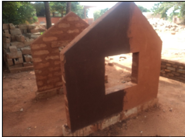
Figure 20. Wall after application of the body of the coating.
