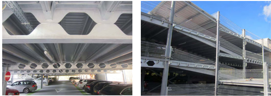
Figure 1. Applications of cellular beam with sinusoidal openings.
