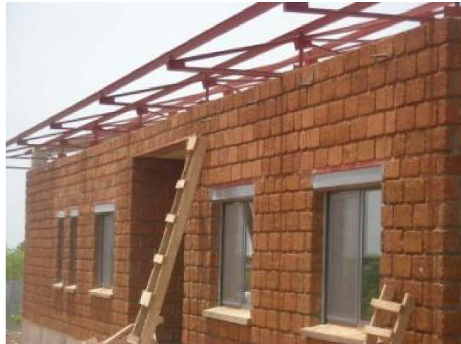
Figure 1. Masonry construction - lateritic blocks - Dano (PN) [4].
