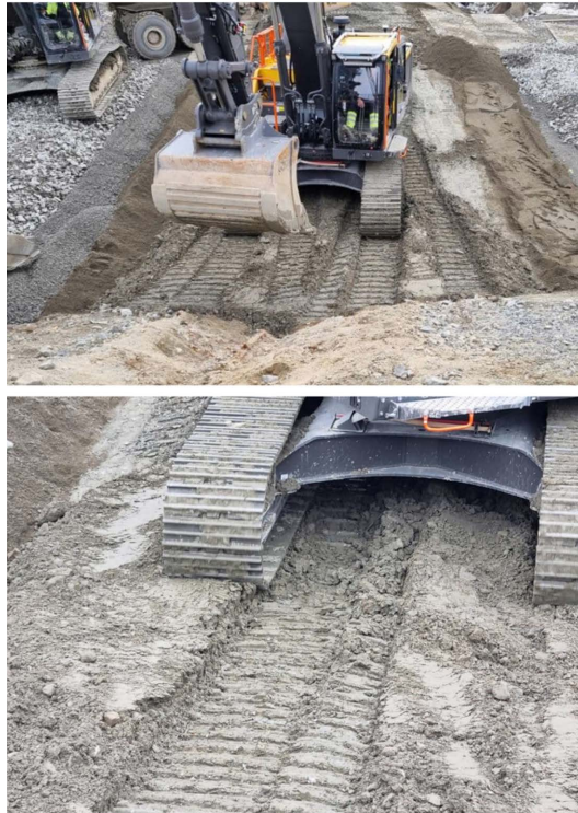
Figure 7. Application of Wet compaction of glacial till to the core zone.
