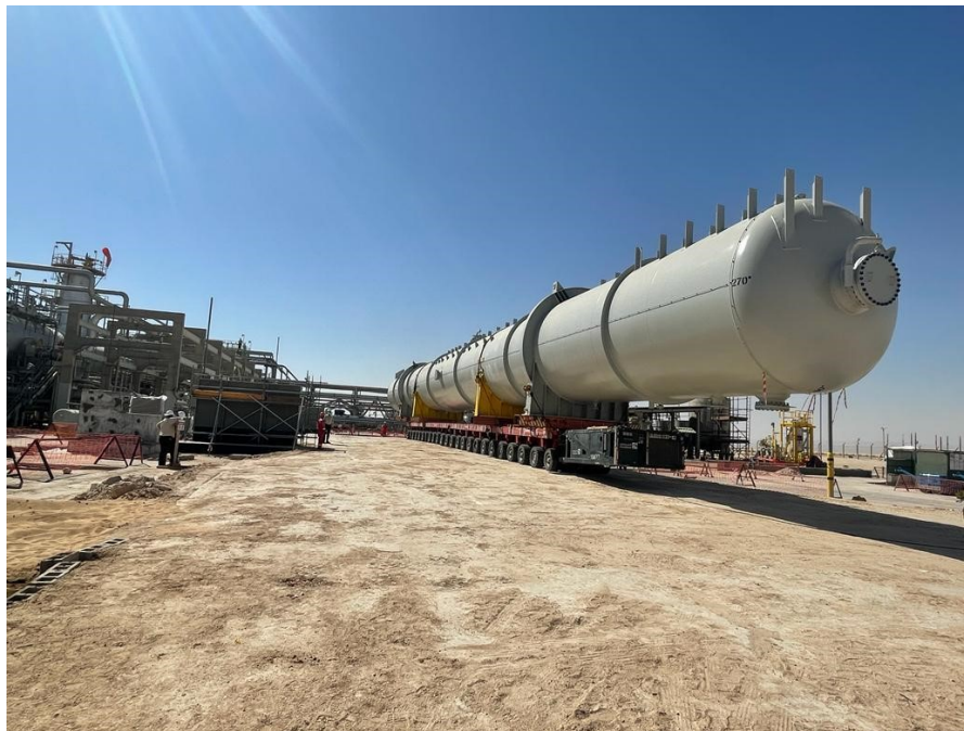
Figure 2. Vessels onboard an SPMT being transported through an operating facility.
