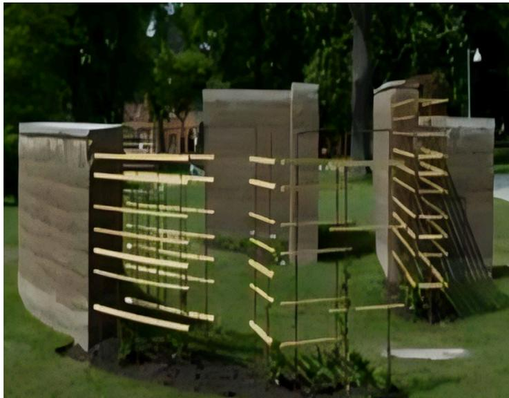
**Figure 2.** Bamboo reinforced rammed earth wall (figure copied from [24]).
