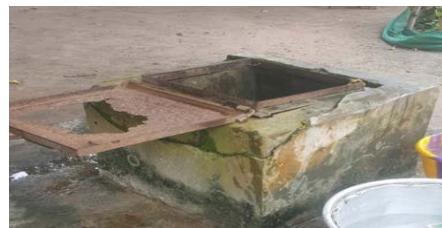
Borehole MF1 water sampling location
