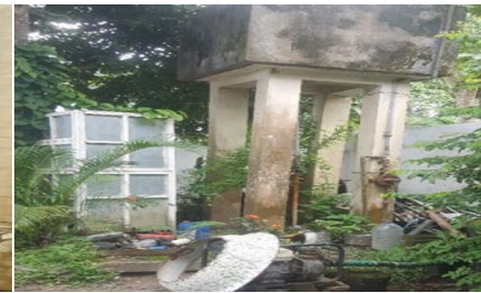
Borehole MF2 water sampling location
