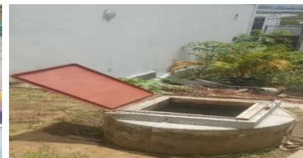
Borehole MF2 water sampling location
