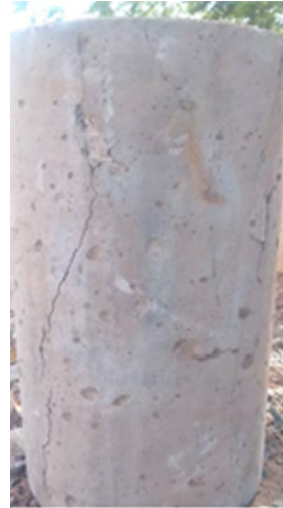
Figure 7. Type of rupture obtained in the cylinders after compression resistance test.
