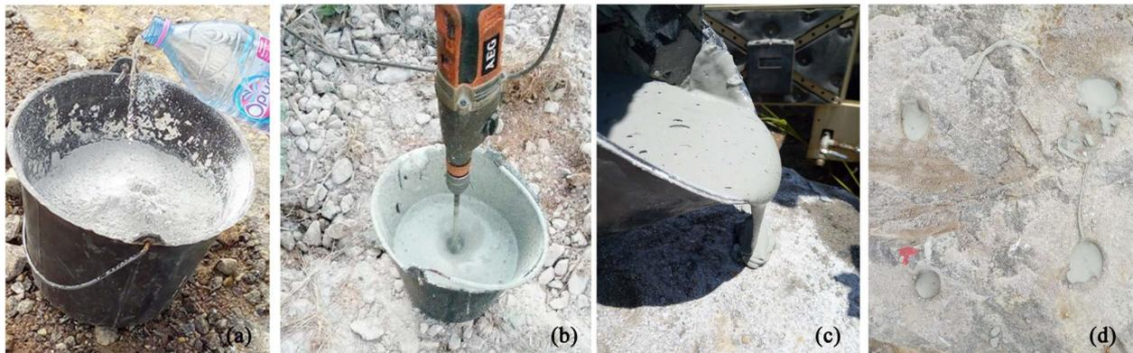
**Figure 3.** Steps of the NEEM mixture process. (a) Adding water in NEEM powder; (b) Mixing; (c) Pouring into predrilled holes; (d) Holes filled with NEEM.
