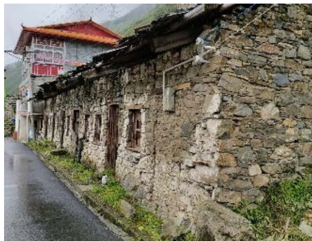
Figure 7. Stone and wood buildings built in the Qing Dynasty in Sermi Village (source of the picture: the author shot).
