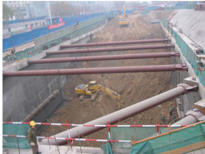
Figure 2. Construction site drawing of open excavation method.
