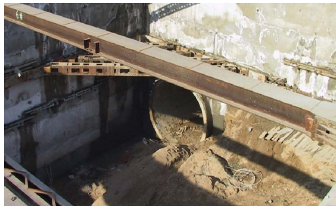
Figure 1. Construction site drawing of open excavation method.
