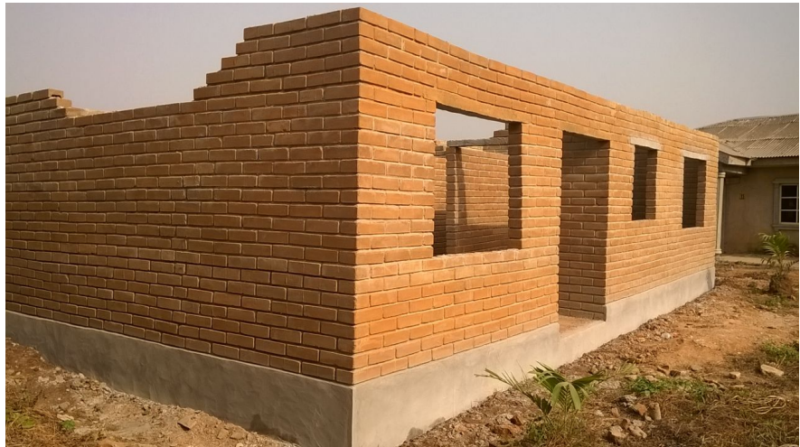
Figure 3. Stabilized interlocking clay bricks used in construction.
