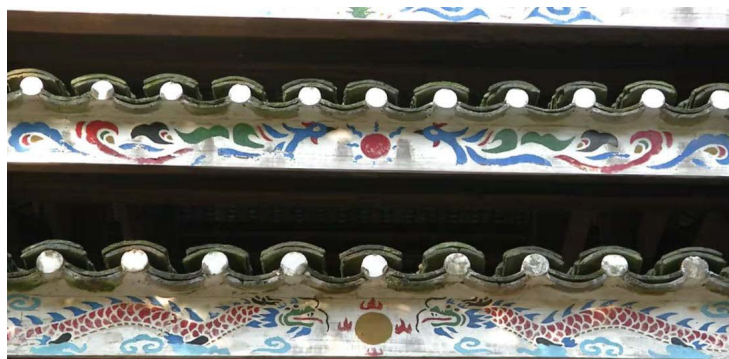
Figure 2. Horse Fat Drum tower cornice.
