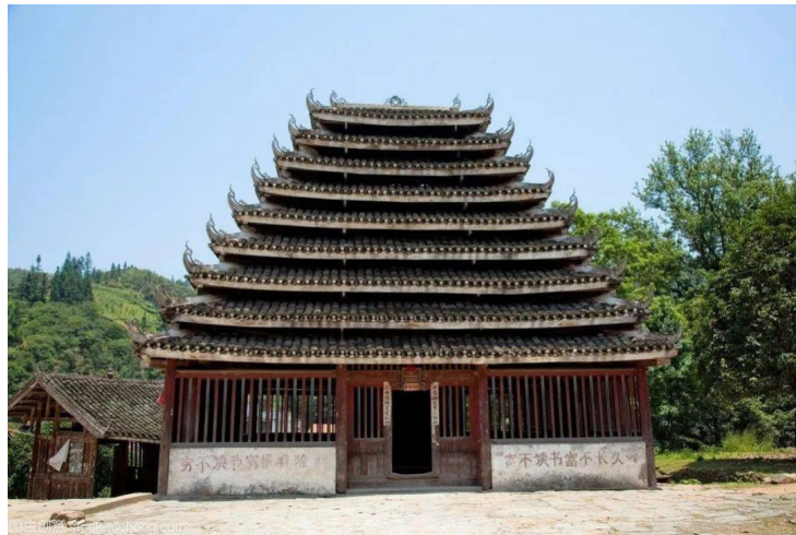
Figure 1. Front view of Ma Fat Drum tower.
