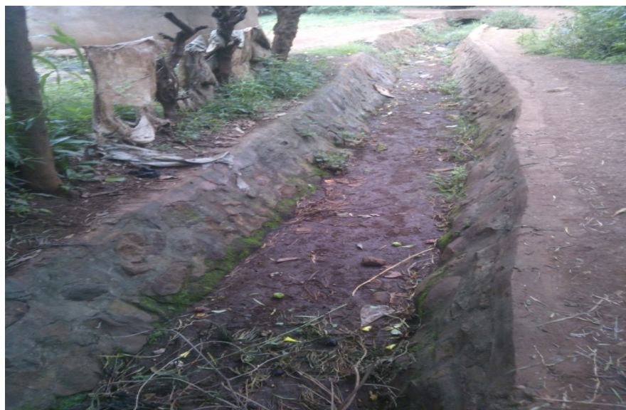
Figure 1. Sample drainage constructed with trapezoidal and rectangular with pitch lining.
