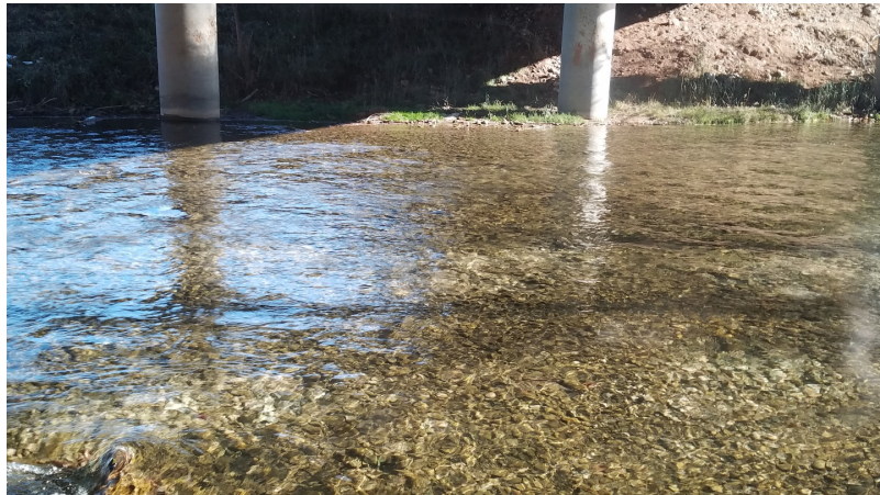
Figure 15. Photo of redds under highway 14 bridge.
