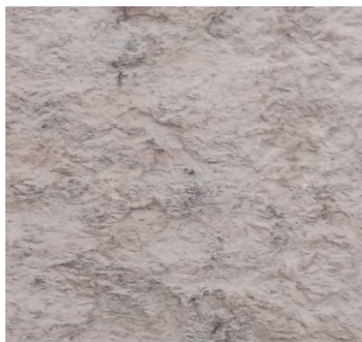
Figure 4. Corrosion, loss, gaps, and Peel off the text hieroglyphic.
