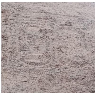
Figure 6. Name of the king suffers from Exfoliation and fragmentation.
