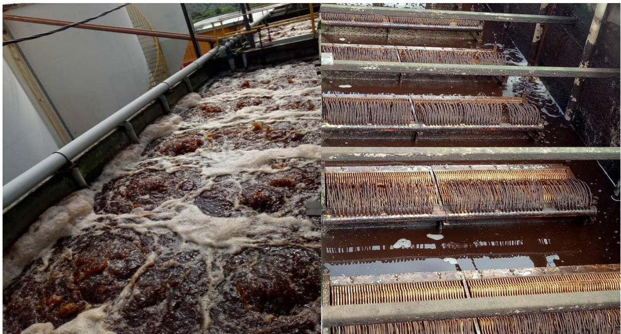
Figure 5. MBR system for POME treatment in palm oil mill.
