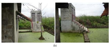
**Figure 4.** Experimental septic tanks in plastic polyethylene at Ahouansori Towéta (a) and ecological above-ground watertight pit latrine in swampy environment of Agla in Cotonou (b) (Photos: H.S. Totin Vodounon, August 2019).
