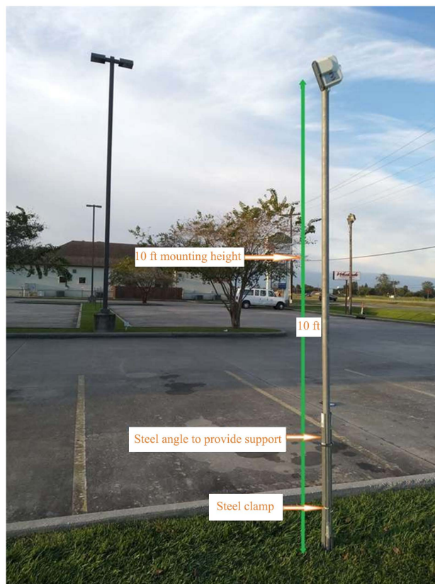
Figure 3. A successful installation of camera.
