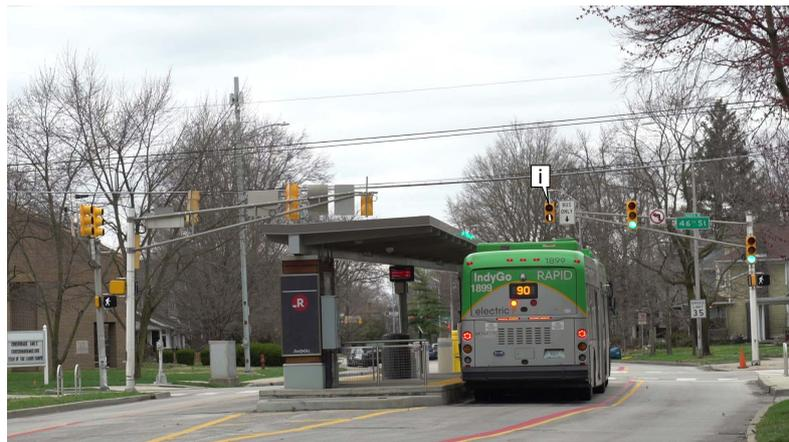
Figure 5. Intersection with near-side bus station.
