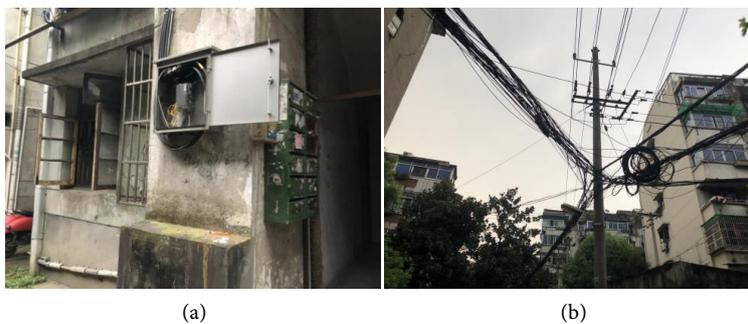
**Figure 5.** Bare electrical accessories and messy cables.
