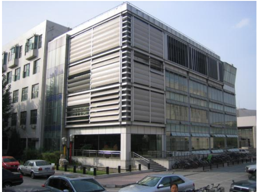
Figure 8. Outer wall of low energy demo building of Tsinghua university.
