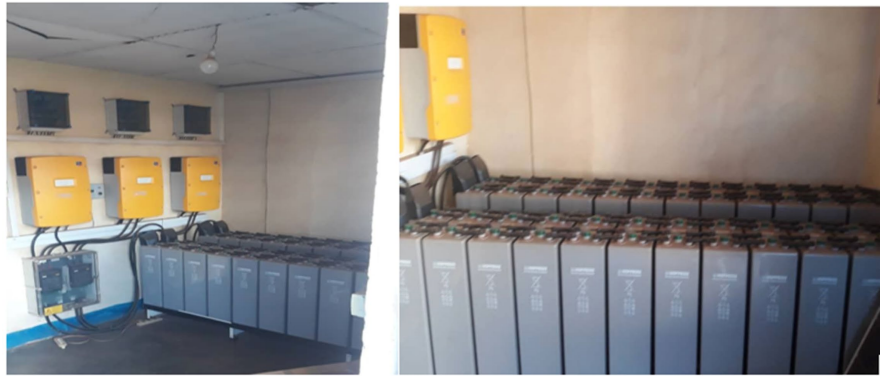
Figure 1. Photo of the battery storage site for the PV system installed at Bugendana Parish.
