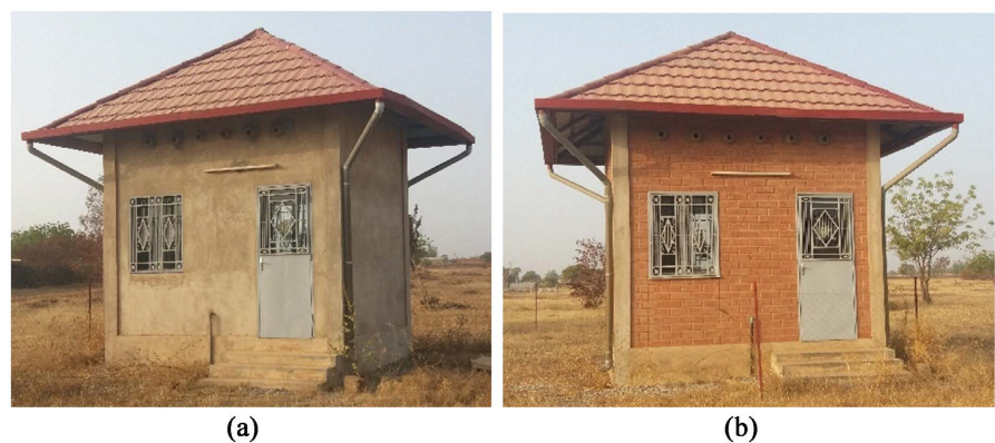
Figure 1. Experimental pilot buildings in cement block (a) and CEB (b) at the 2iE Kamboinsé/Ouagadougou.
