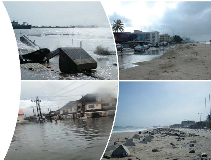
Figure 3. Flooding of the bar beach and the surrounding areas adjoining beach in Victoria Island Lagos on 29 the May 2009.
