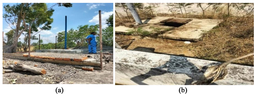
Figure 7. Different Placenta Pits in Healthcare Facilities. (a) HCF Standard Placenta Pit (Nkasi DC Hospital); (b) HCF Defective Placenta pit without a Lid (Laela HC)
