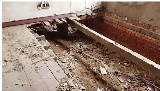
Figure 9. The foundation of the school.
