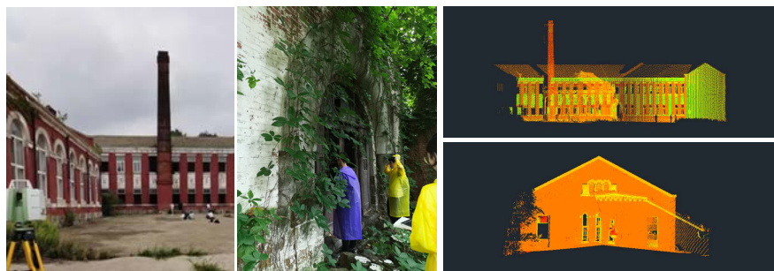
Figure 4. Building status mapping and point cloud data collation.
