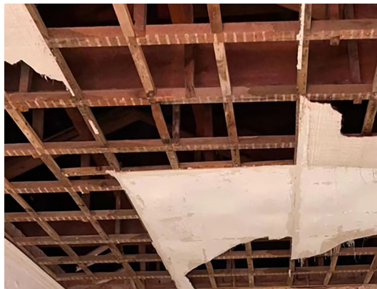
Figure 11. The roof structure of the school.
