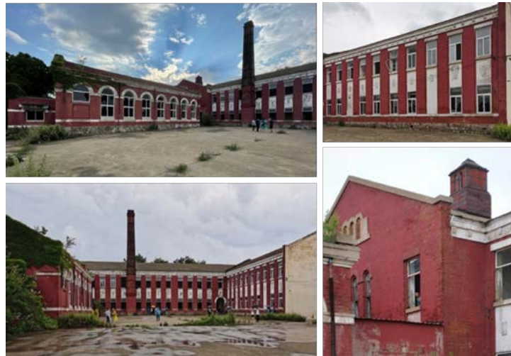
Figure 3. Status photo of the site.
