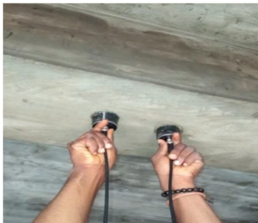
Plate V: Tested point on first floor beam.
