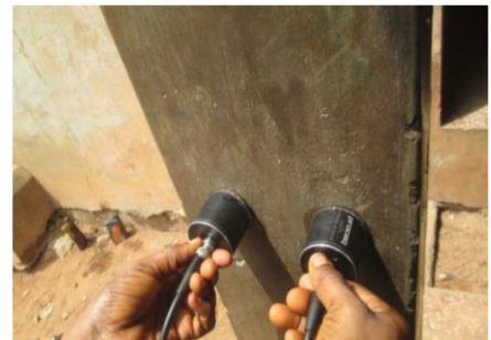
Plate VI: Tested point on a ground floor column.
