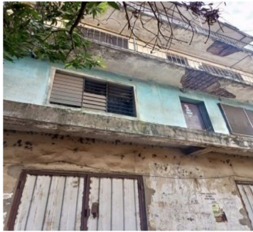
Plate I: Left hand side view of the tested building.
