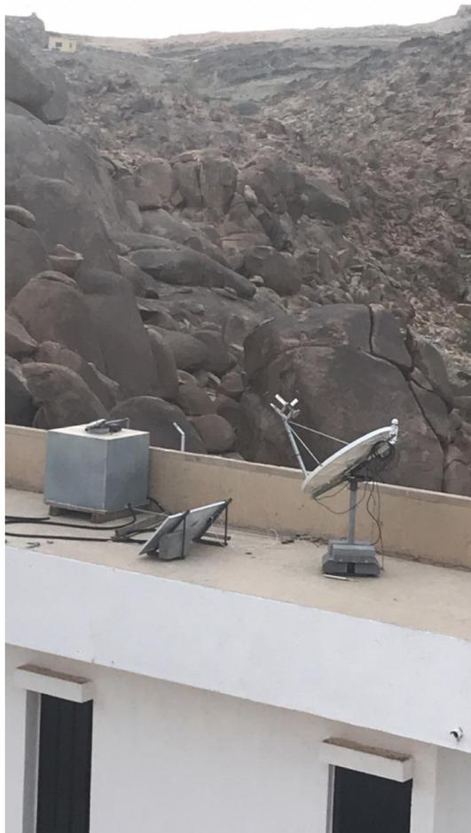
**Figure 6.** A photo of a complete seismic monitoring station (strong motion station) that was established on the body of the Tandaha dam.
