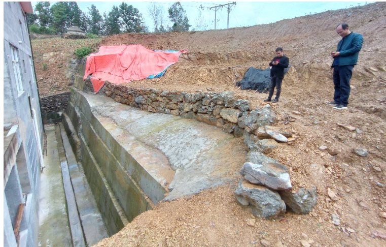
Figure 6. Image of a group of landslides in Huaishu village after treatment.
