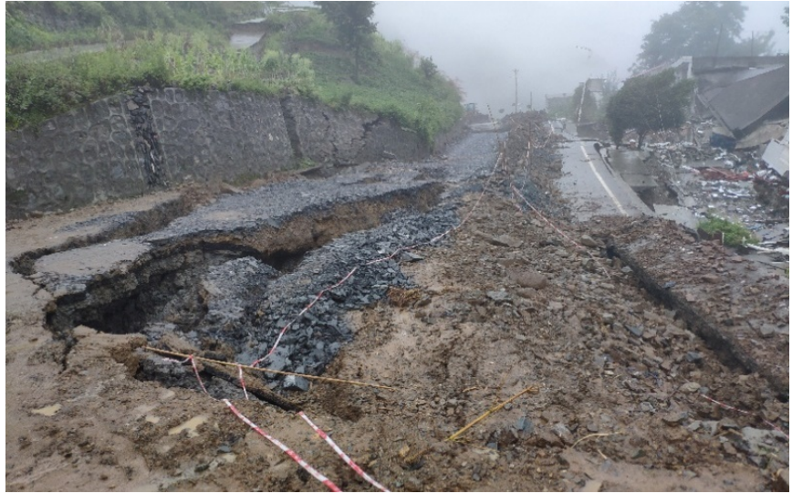
Figure 8. Traffic interruption due to landslide in Group 4, Zhujiexi village.
