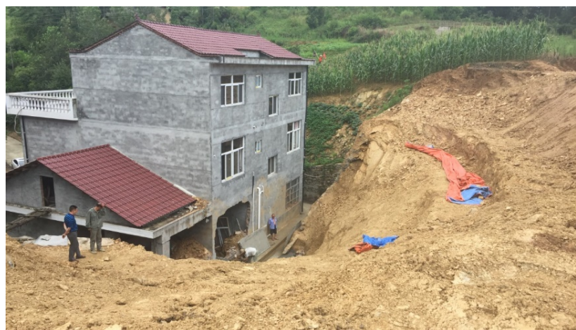
Figure 5. Image of Group I Landslide in Huaishu village before treatment.
