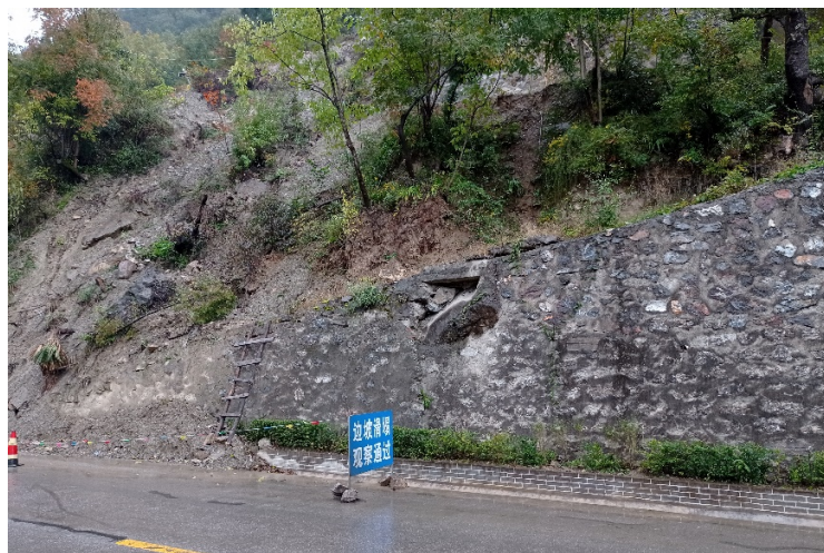
Figure 7. Landslide road blocking in Guandi mountain village.
