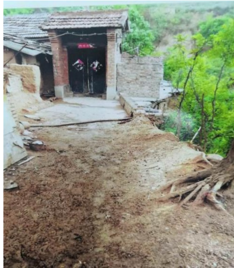
Figure 3. Image before the landslide behind the white building in the building materials factory.
