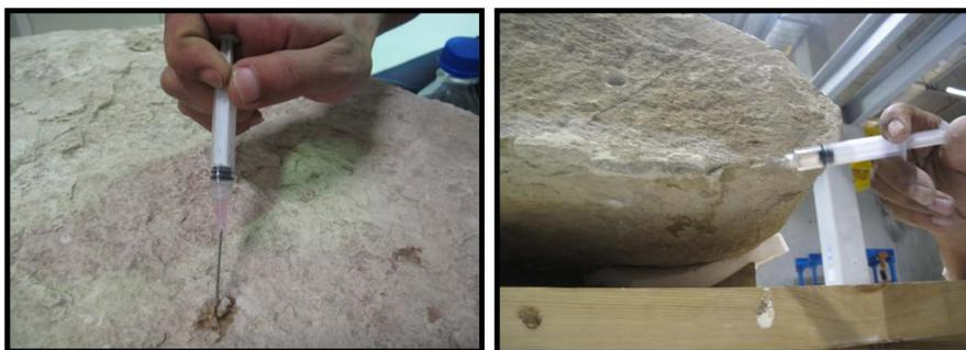
**Figure 24.** Consolidation of the weak points of stone edges.
