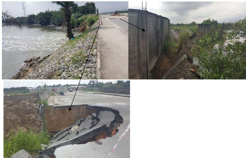
**Figure 6.** Failures due to erosion of bridge abutment at Nkpgogu.
