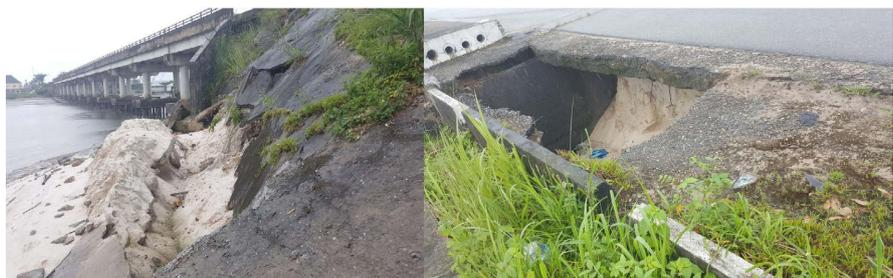
**Figure 5.** Erosion of Abutment base and failure of asphaltic surface.
