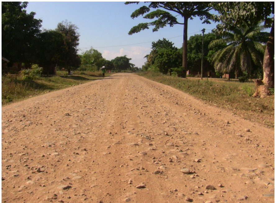
Figure 1. Typical gravel road; study road (2021).
