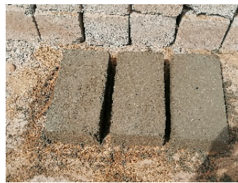
Figure 7. Mortar of cinder block (Building site).
