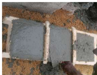
Figure 9. Building site concrete.
