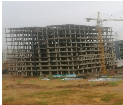
Figure 2. CORIS BANK building in area ZACA.
