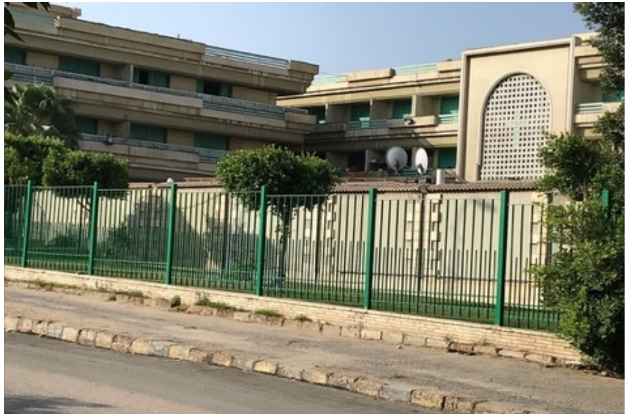
Figure 10. Influential structures occupying the pavement and narrowing the road; the author, 2020.
