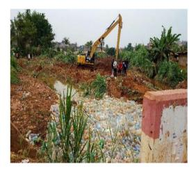
**Figure 17.** Plastic waste pollution at Biyem Assi. Note the Caterpillars and city council workers widening the valley width to facilitate water circulation. Source: Ojuku, 2020.
